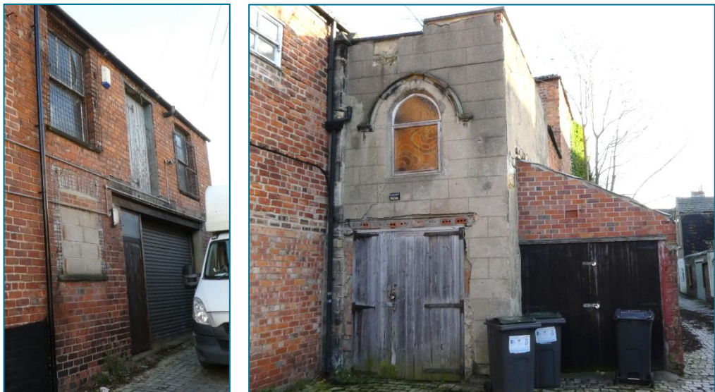
Left: Outbuilding with hoisting door. Right: Various brick and rendered outbuildings along the longer back lane. The central one is Tallyman's Cabin; it used to be crenelated and has a Neo-Gothic entrance behind the abutting brick garage. (Photos © Gaby Rose, November 2023)
