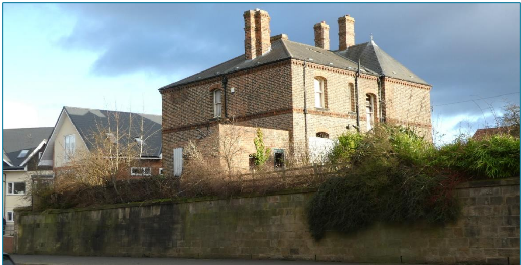
C6 – Top : Semi-detached houses along Houghton Road possibly dating from the 1930s, with unusual front extensions. Centre : The terrace of former railway housing appears little altered. The modern building to the right is of no interest. Note the former higher road level. Bottom : The Vicarage to St James church is currently derelict. The tall retaining wall originates from the later lowering of the road. Note the incongruous modern development in its immediate surroundings to the left/east. (Photos © Gaby Rose, February 2024)
