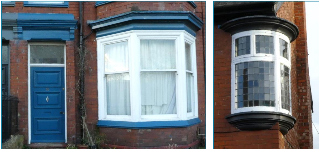
Left (Photo © Gaby Rose, November 2023): Original panelled door with stone canopy over and old sashes along North Lodge Terrace. Right (Photo © Gaby Rose, December 2023): Curved first-floor window with leaded glazing along Elmfield Terrace.
