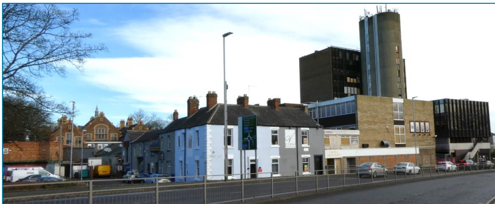
G – View across the inner ring road looking northeast. The corner building (Holly Street and nos. 8-9 Kendal Street) is the oldest surviving heritage asset in this area. In the background, the attached, slightly lower building to the left/north includes the 1879 Quoit Club inscription, in the approximate location of the yellow van. Behind it, [H] Central Secondary School within the Conservation Area under review can be glimpsed. Northgate House to the right/east is completely out of scale and not in keeping with the surrounding architectural language. (Photo © Gaby Rose, February 2024)
