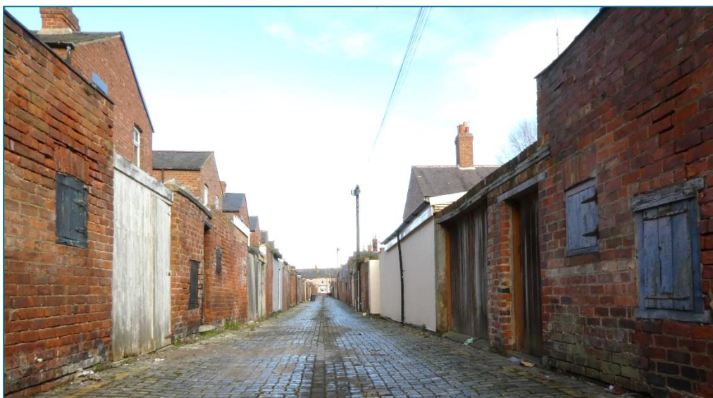
F – Back lane to rear of North Lodge Terrace, looking north; note the original shuttered openings to both sides. The rendered wall further on to the right/east has a harmful impact on the historical character of this lane. (Photo © Gaby Rose, February 2024)
