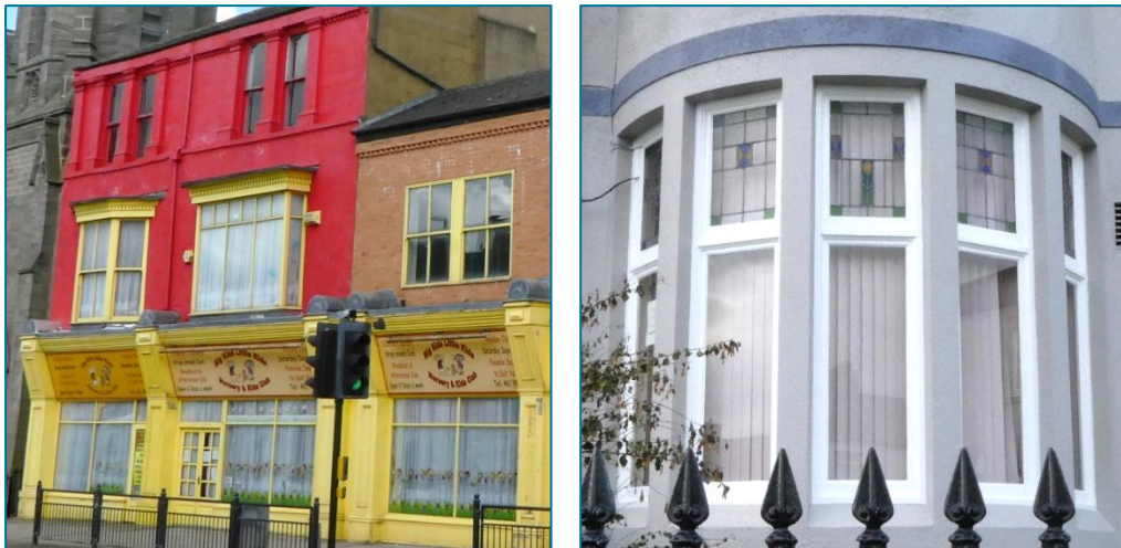
Left (Photo © Gaby Rose, August 2023): Traditional windows with slim frames and glazing bars and a traditional-style shop front were provided under the 2002-05 Northgate HERS. Right (Photo © Gaby Rose, December 2023): Coloured glass with lead glazing bars were restored under the 2005-09 Northgate PSCA (see section 3.6).
