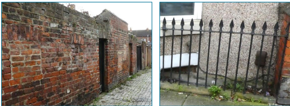
Left: Scoria-paved back lane off McNay Street lined with original rear-yard walling including openings, the coal holes now blocked. Right: Original metal railings set in stone in front of basement along Station Road. (Photos © Gaby Rose, November 2023)
