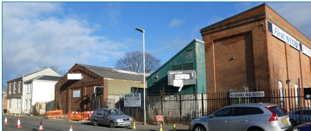
A3 – Top : Formerly the Globe, now flats; the attached building is modern. Bottom : The former water tower is the brick building to the right/south, its tank now removed and a new roof provided. Attached to it is one of the timber structures shown on the 1939 map. The brick building to the left marks the northwest corner of the former Locomotive Works and, like the water tower, has recessed panelled brick walling. (Photos © Gaby Rose, February 2024)
