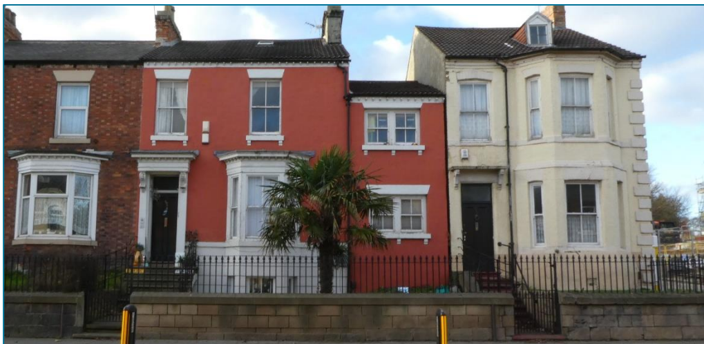
Top (Photo © DBC, before July 2001): Nos. 105 (grey) and 109 (end property) High Northgate prior to works. No. 105 including its boundary wall was improved under the 2002-05 HERS, and No. 109 under the 2005-09 PSCA, both receiving new metal railings. Bottom (Photo © Gaby Rose, November 2023): The properties still stand out positively today.
