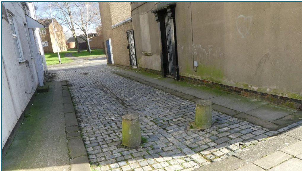
A9 – Top : Nos. 38-70 North Road looking northeast. Centre : The terrace viewed from the north, looking southeast. Bottom : Scoria-paved lane with worn stone kerbing; also note historical door surround to the right/east, at no. 70. (Photos © Gaby Rose, February 2024)
