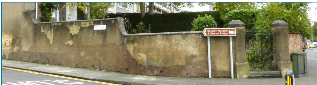
Top left: Back lane with scoria and sandstone block surfacing. Top right: Ornate, cast-iron railings on top of ashlar stone/brick boundary walling between private front garden and public realm. Bottom: Rendered garden wall on street corner with stone copings and prominent gate piers. (Photos © Gaby Rose, November 2023)
