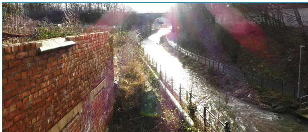
B – Top (Photo © Gaby Rose, August 2023): Albert Road Bridge viewed from the footpath along the Skerne, looking north, with the original structure partially concealed behind the later one. The Council has agreed to paint the bridge railings, at the request of the Friends of the S&DR, to enhance its appearance for the 2025 S&DR bicentenary 236 . The ruined brick building is to the right/east. Bottom (Photo © Gaby Rose, February 2024): View from Albert Road Bridge (through mesh panelling) with the brick building to the left/east and [7] Skerne Bridge in the background. Note the traditional railings on the left-hand/eastern riverbank.
