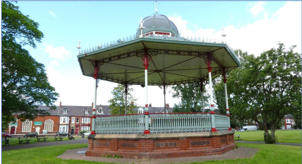
[9] Bandstand to West of Bowling Green (photo © Gaby Rose, July 2023): Restored and re-opened in 2010 after long-term dereliction. North Lodge Terrace in the background.
